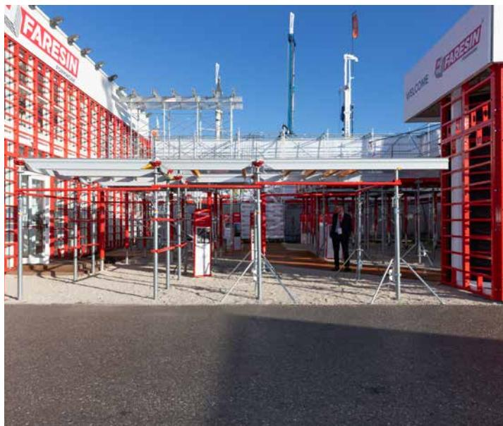
**FLEXI DECK** is an easy-to-use slab formwork system that can be moved manually and, thanks to the **dropping heads**, allows for the **early dismantling** of beams and planking used in the casting phase.
